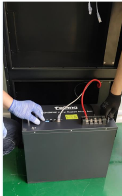
2. Connect the communication cable. 3. Set the battery ADD address.
