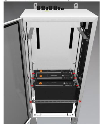
Lock the 6 dowels for these 3 batteries.
